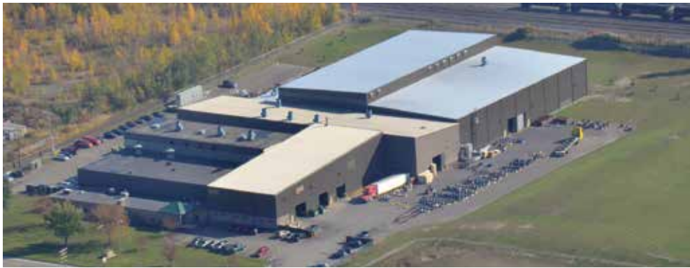
An impressive aerial view of the recently expanded McInnes Rolled Rings plant.
